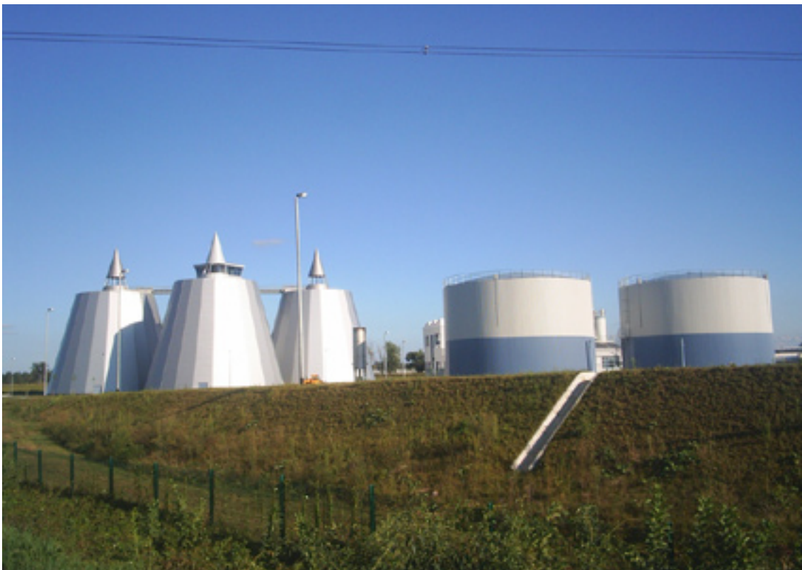
The Zagreb wastewater treatment plant has been criticised for offering poor value for money. Photo: UZOR
