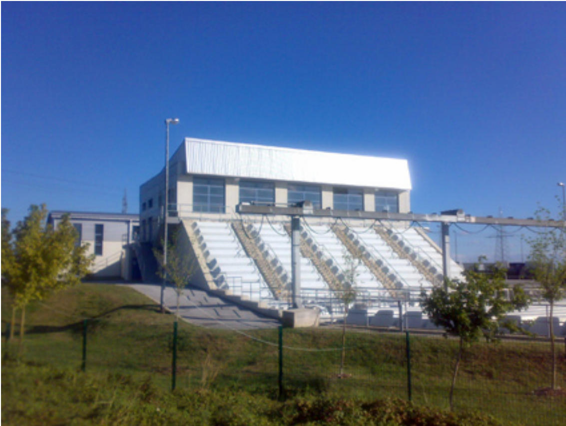
Zagreb wastewater treatment plant. Photo: UZOR
