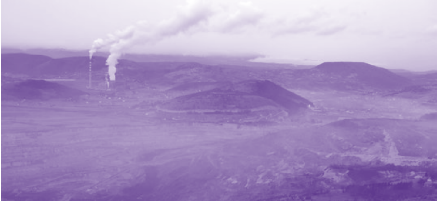
▲ The Pljevlja plant and mine
