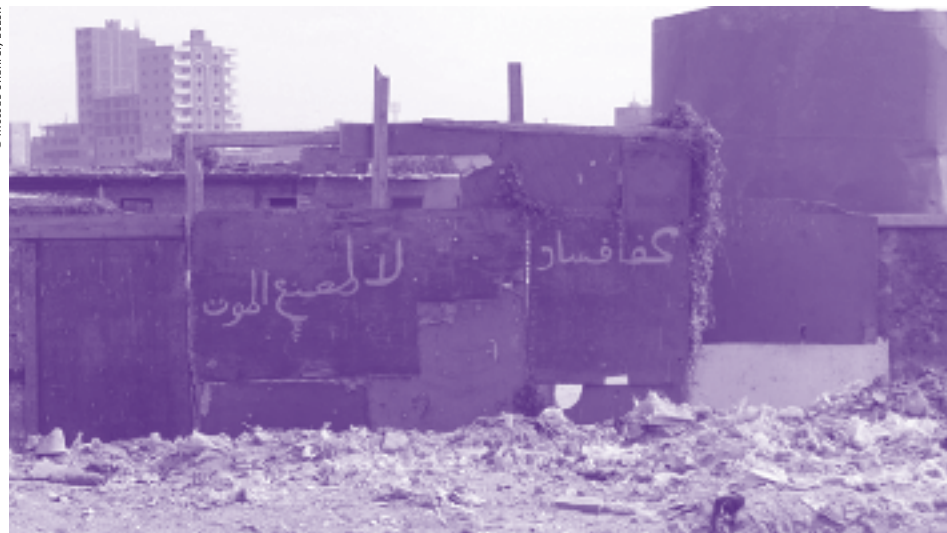
▲ Graffiti in the ERC project area, saying in Arabic "Enough corruption", "No to the factory of death".
